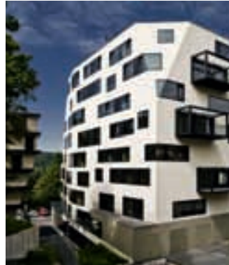
Triplex - residential building, Karlovy Vary
